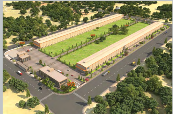
Jaipur Plant, India
